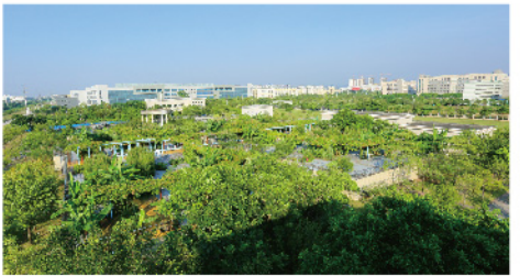
市政污水处理案例 采用立体生态处理技术 MUNICIPAL WASTEWATER TREATMENT PROJECT Multi-dimensional ecosystem technology for wastewater treatment
