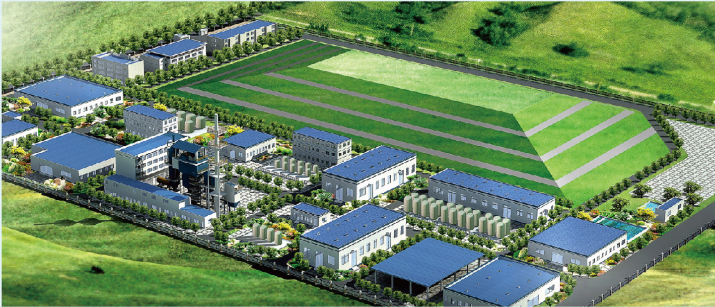
江西工业固体废物处置中心 承担了全江西省工业、社会危险废物的集中处理处置，可处理31类危险废物， 包括资源化利用，物化、焚烧、固化处置等。 JIANGXI INDUSTRIAL SOLID WASTE DISPOSAL CENTER Responses for disposal of industrial and household hazardous waste for entire province, qualified for 31 category of hazardous waste including resource recovery, physiochemical, incineration, stabilization and solidification.
