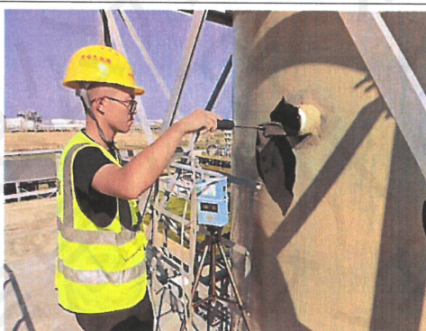
焚烧废物丙类仓库废气排放口 DA003
